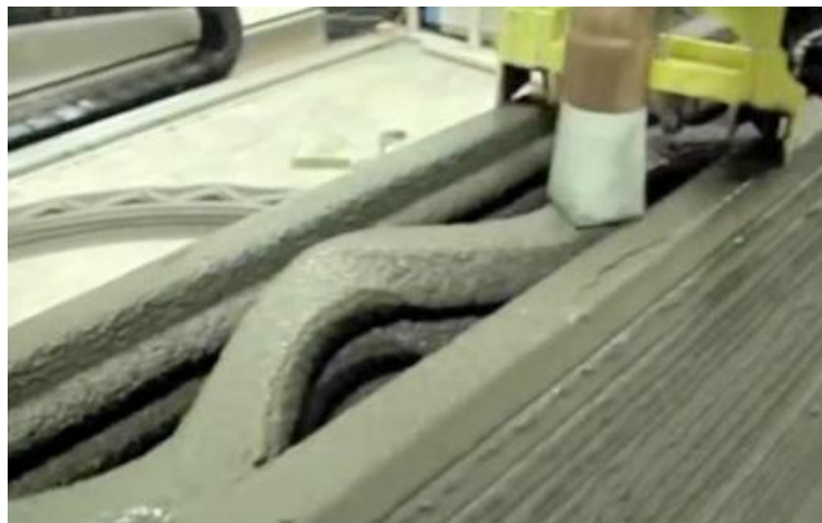
Fig. 26. Contour Crafting Nozzle extruding concrete ( University of Southern California, 2014 )
