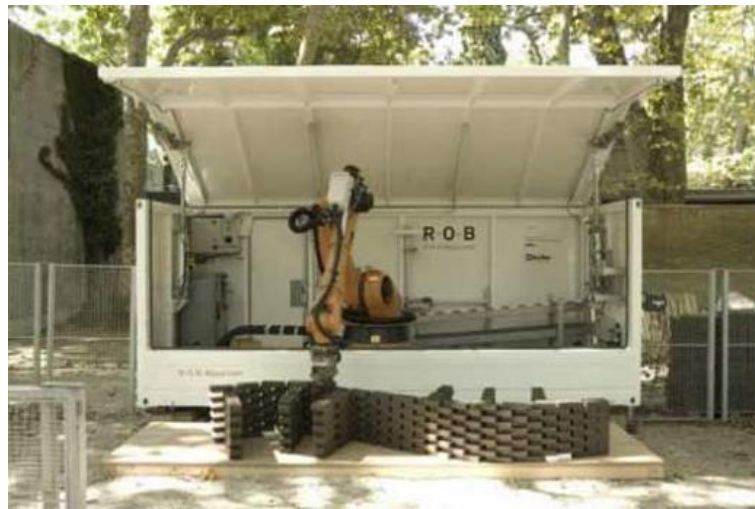
Fig. 23. R.O.B., deployable robotic arm to build architectural elements on site. (ETH Zürich with Gramazio & Kohler, 2008)
